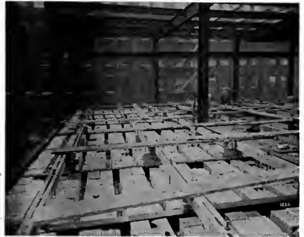
VIEW SHOWING CONSTRUCTION OF FLOOR ARCHES
